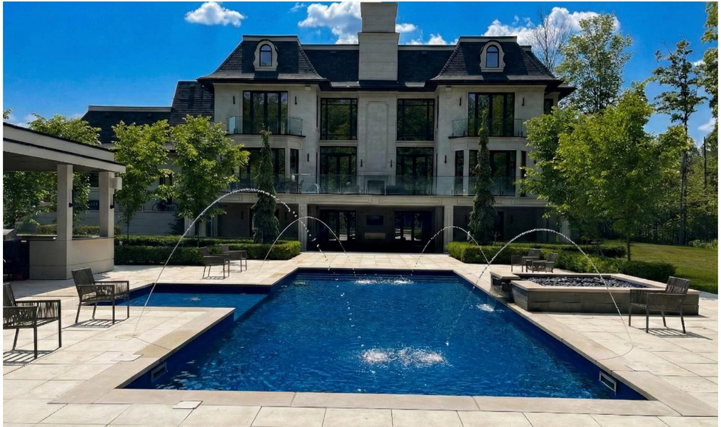
This Burlington pool and landscape project features a 16x38 rectangular vinyl liner pool with full size stadium style stairs, a 10x12 sunledge and an integrated 8x8 hot tub. Also featured were 4 laminar deck jets and 2 bubblers. The patio is 24x24 porcelain tile and the pool coping is 12 inch limestone. The landscaping included over 600 plantings, 50 trees and automated lighting and irrigation systems.
